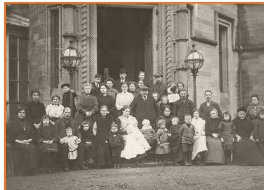
1914 Sillerbeth Hall. Hawick, Scotland.
